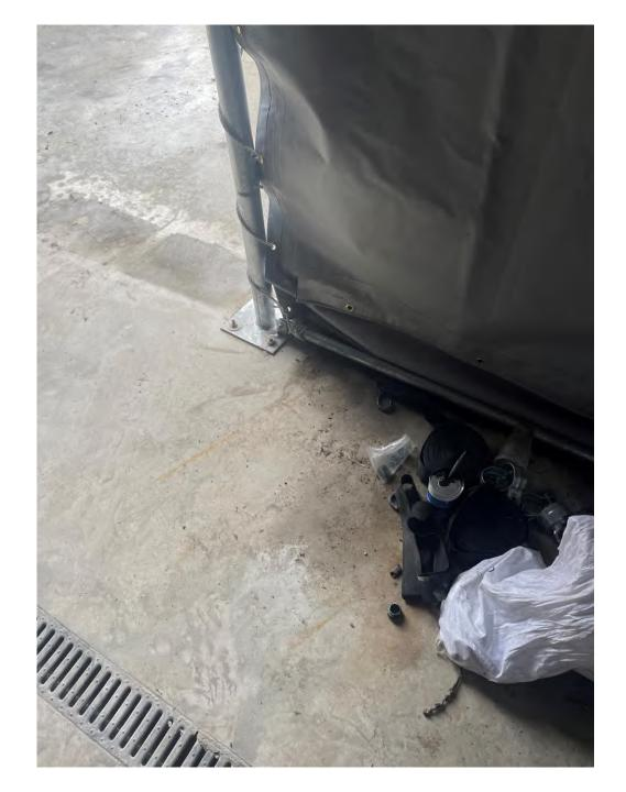
Image to show the unauthorised structure is affixed by bolts to the hardstanding.
